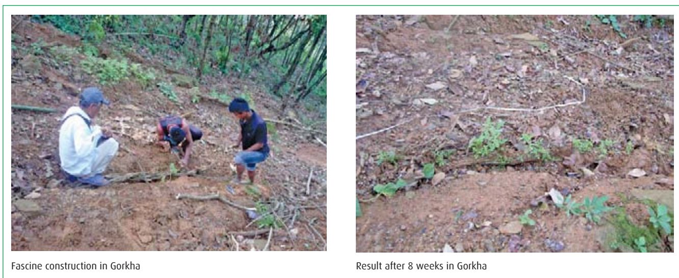
Figure 4: Fascines installed in Budhathum, Dhading and Dhodre, Gorkha
