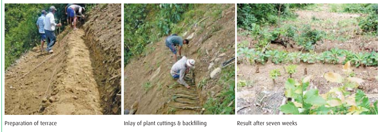
Figure 3: Construction steps of brush layering (Dhodre, Gorkha)
