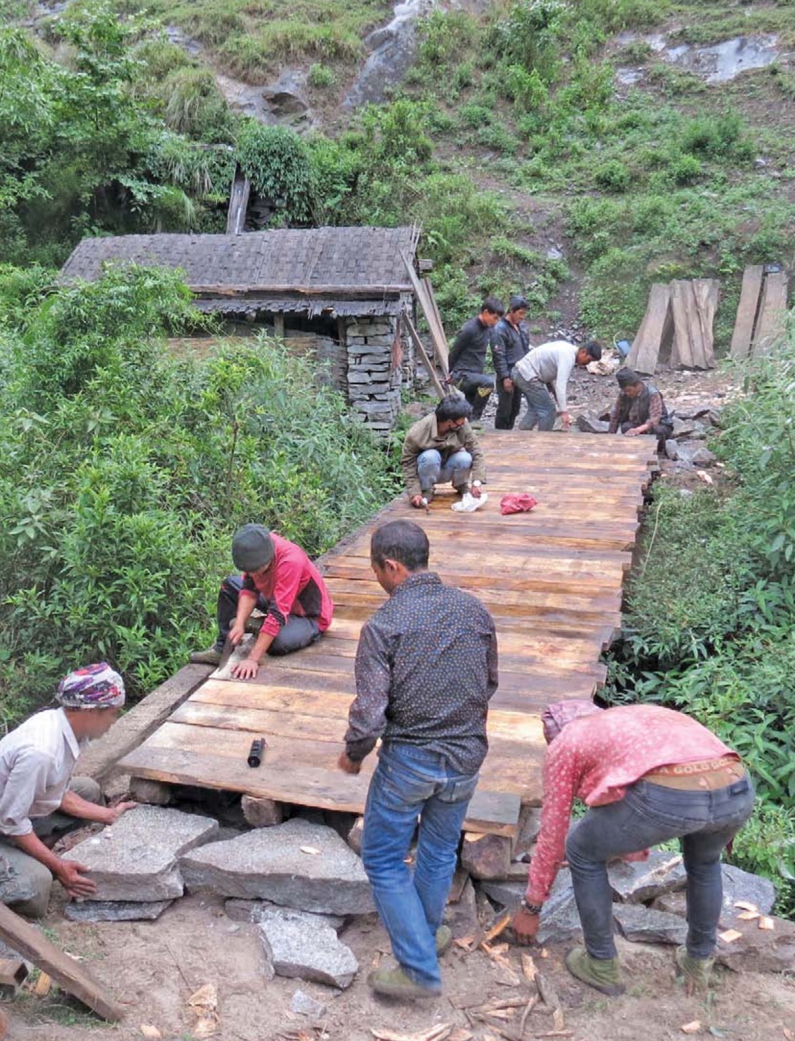
Repairing foot trail bridge at Sirdibas, Manaslu Conservation Area, using local materials. The bridge provides a vital connection for local communities. © National Trust for Nature Conservation, Hariyo Ban Program/Bishnu Singh Thakuri
