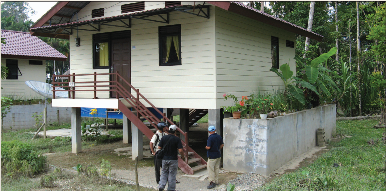
The constructed wetland shown to the right of the house is an example of the household-level wastewater treatment systems that were constructed in Aceh, Indonesia, after the 2004 Indian Ocean tsunami. The constructed wetland is part of the water and sanitation system that was built by the American Red Cross. Both the house and the treatment wetland were elevated for protection against flooding. The floor of the treatment wetland is sealed to prevent wastewater from contaminating the groundwater before it has been treated. The house was constructed by the British Red Cross and uses timber that has been certified by the Forest Stewardship Council. © Azhar/WWF
