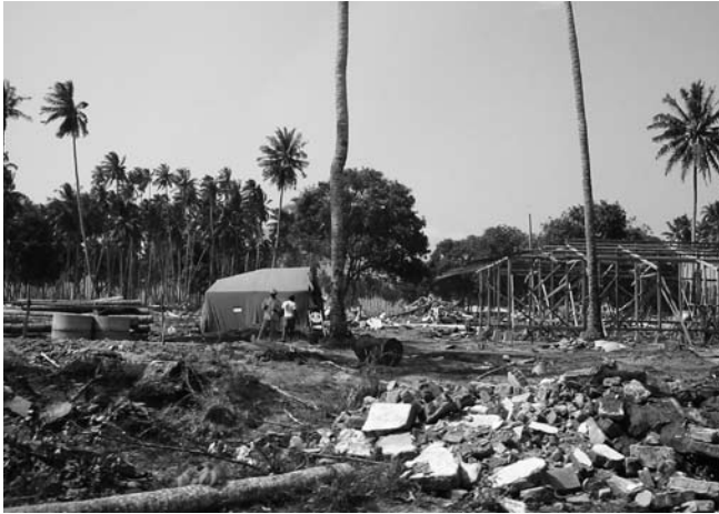
Residents rebuilding after the 2004 tsunami, Banda Aceh, Indonesia
