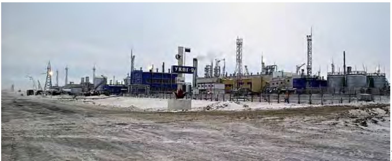
Gas treatment unit No.9 at Kharvutinskaya area of Yamburg field.
