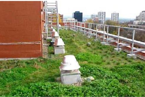
**Above:** *Eceroofs replace conventional roofing with a living, breathing vegetated roof system. This type of roof significantly decreases stormwater runoff, saves energy, reduces pollution and erosion, and helps preserve fish habitat.*
